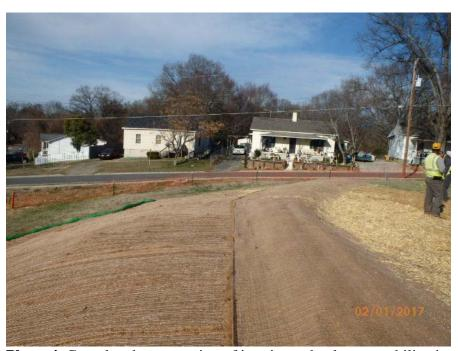
Photo 4. Completed construction of interim embankment stabilization on-site.
