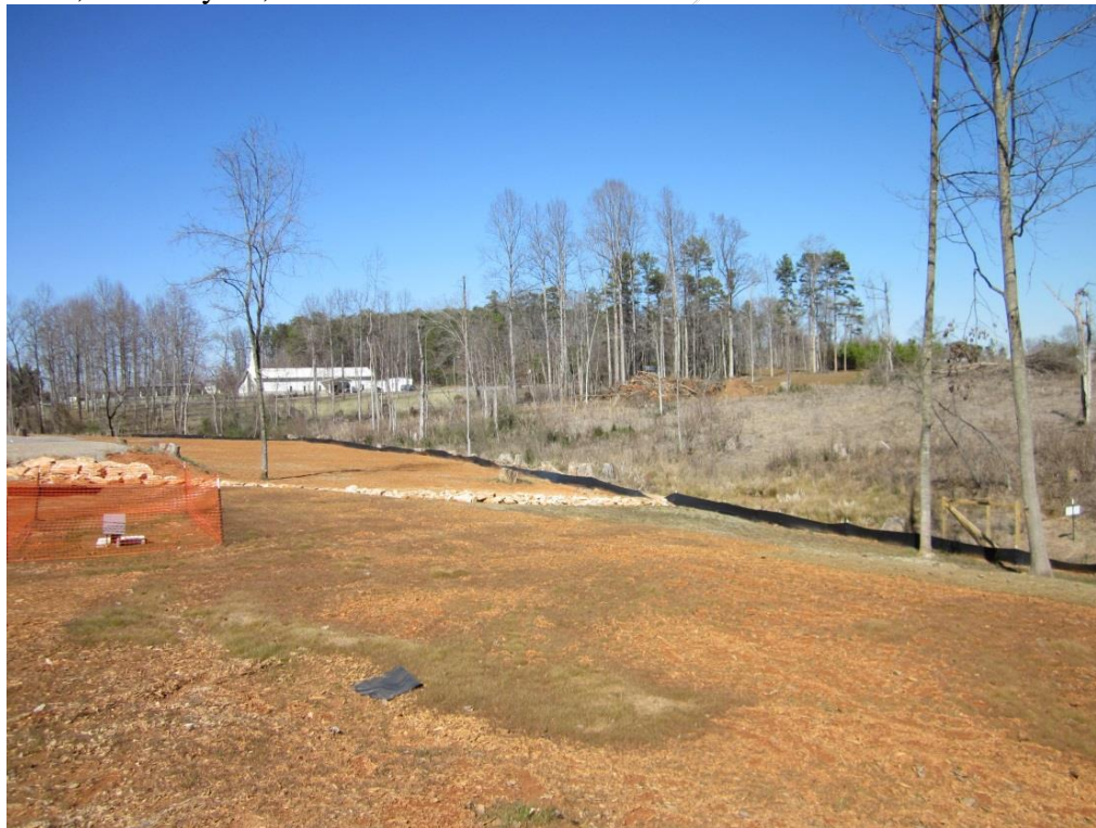
Photo 4. Looking north over the excavated section of site backfilled with clean topsoil. Source: DPH, February 28, 2012.
