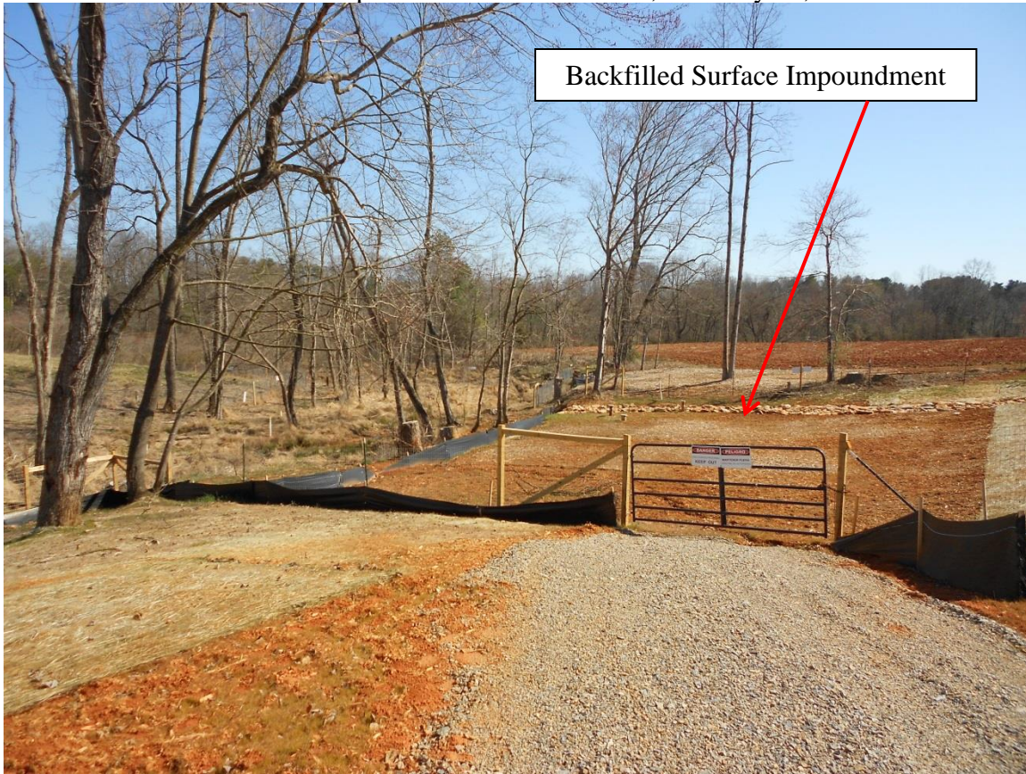
Photo 1. Backfilled surface impoundment. Source: DPH, February 28, 2012.
