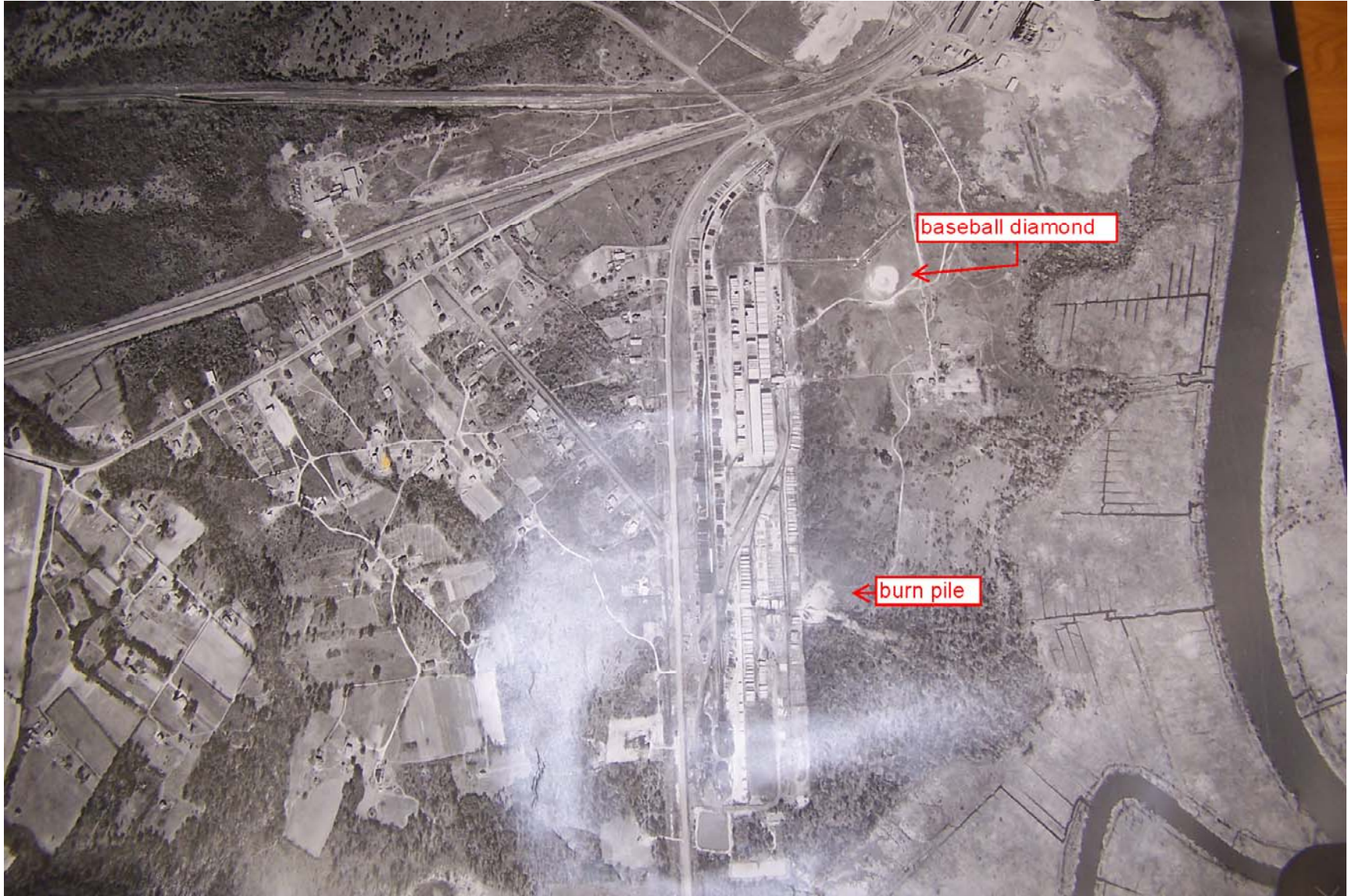
Photo 14. Site areal photograph provided by a community member on October 14, 2010. Photograph was labeled “1965”. Note the location of the baseball field and the area that was identified as the location of a treated wood burn pile.
