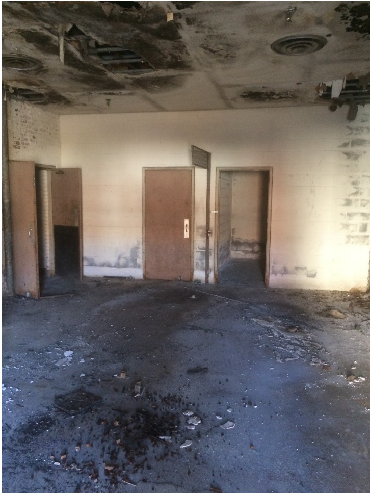
Photos 1 & 2. Evidence of deteriorating ceiling and falling debris in Building No. 2. Source: DPH, October 25, 2016.
